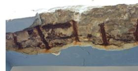
Figure 1 :: Spalled Beam element
