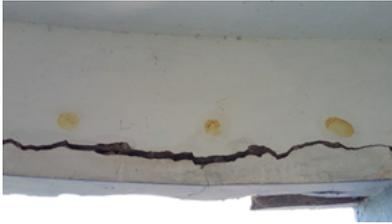
Figure 2 :: Crack in the Tension zone of a beam
